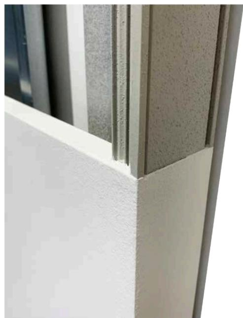
The counterframe includes constructive details, such as the innovative resin-coated profiles, that can easily be painted or decorated to match the wall and make the structure completely invisible and integrated into the wall, for a perfect camouflage of the structure.
